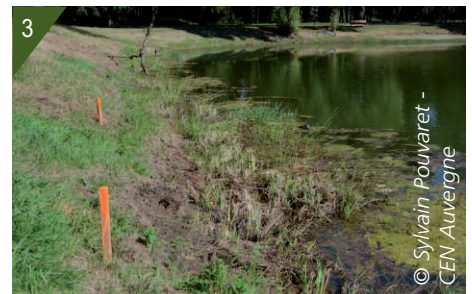
2. A plot prior to the work in September 2011. 3. A plot after the work in August 2012.
