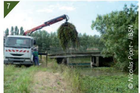
6. Manual uprooting. 7. Mechanical uprooting.
