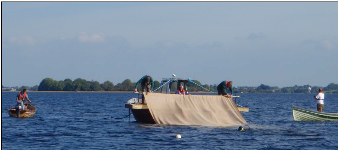
Figure 22: Large-scale geotextile placement operation at Mogan's Bay. The photograph shows a 5 m-wide by 100 m-long roll of geotextile being deployed from the boat.
